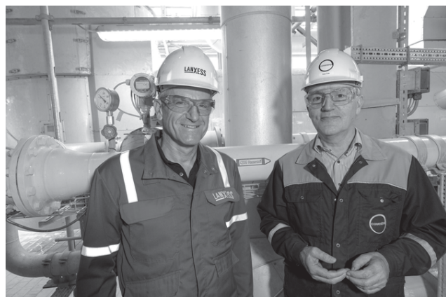
Michael Ertl, Head of LANXESS' Inorganic Pigments business unit, and Rob Eek, Production Manager at Covestro in Krefeld-Uerdingen, stand in front of the new hydrogen pipeline serving LANXESS' iron oxide plant.
